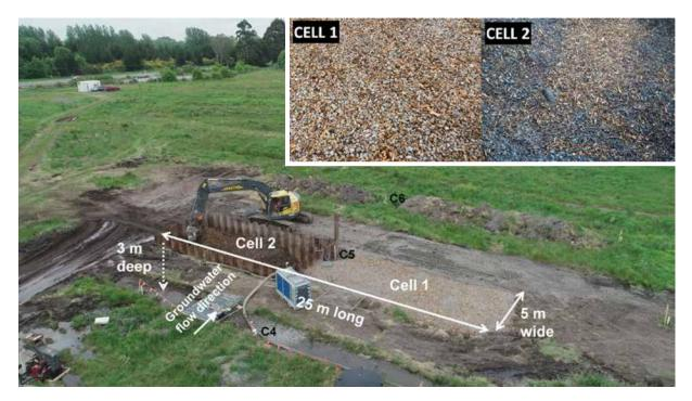
**Fig. 14.** / Pictures of the 50/50 woodchip/gravel mixtures that make up the denitrification wall, and a showing installation works. Cell 1: chipped wood mixed with 20-40mm gravel rounds. Cell 2 hogged wood mixed with parent aquifier material, screened of material under 20mm diameter. The positions of monitoring wells C4:C6 are marked on the photo.
